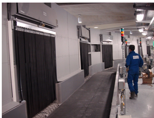
Curtains in security staff zone
